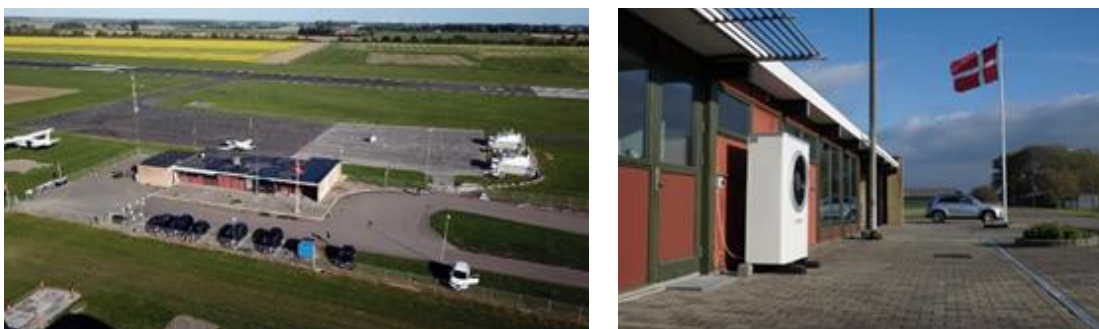
Figure 1.1-1 Aerial photo of the airport and picture of the heat pump installed at the airport.
