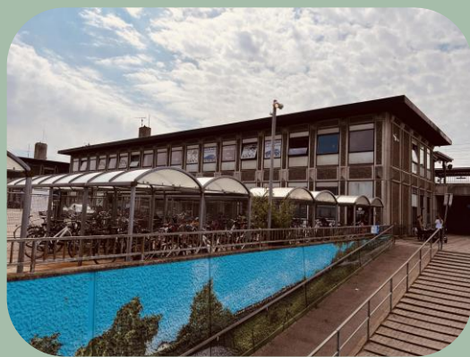
Bicycle parking and tunnel connection
