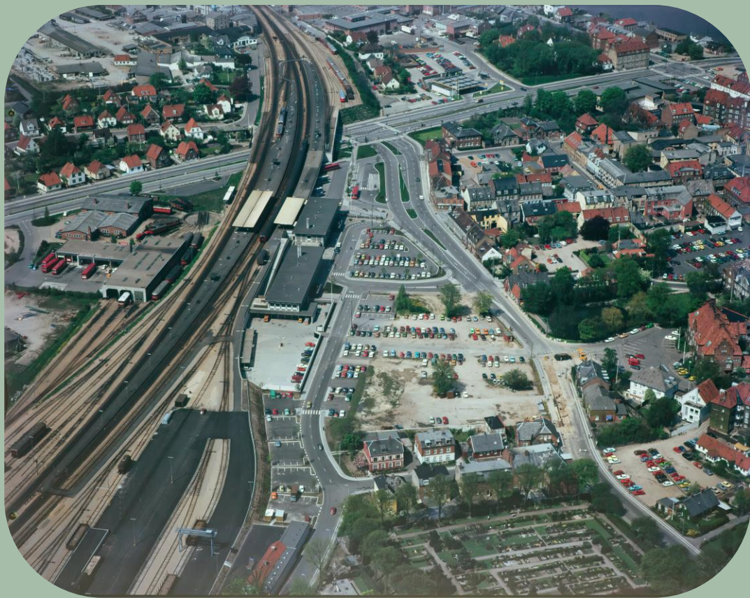
Overview of Holbæk station and immediate surroundings
