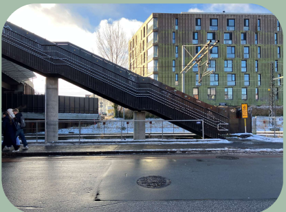
Space under the bridge of the light rail stop
